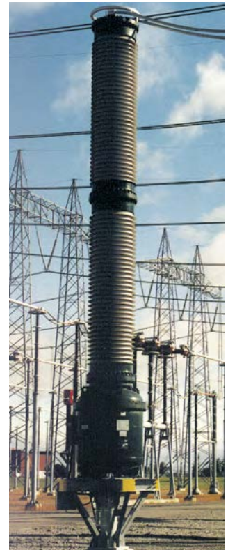
Fig. 4.2-14: 800 kV gas-insulated current transformers
