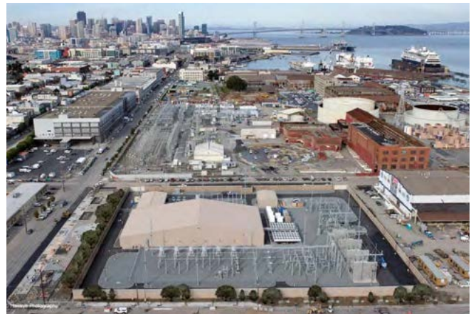
Fig. 2.2-6: Converter station of the TransBay Project close to the city center of San Francisco. The world's first VSC HVDC transmission scheme in modular multi-level converter (MMC) topology
