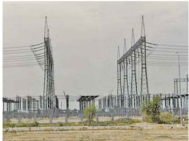
Fig. 3.1-20: One-breaker-and-a-half arrangement, 500 kV, Pakistan
