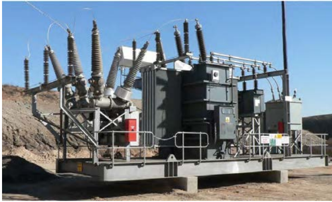
Fig. 2.4-14: 145kV 10MVA skid substation
