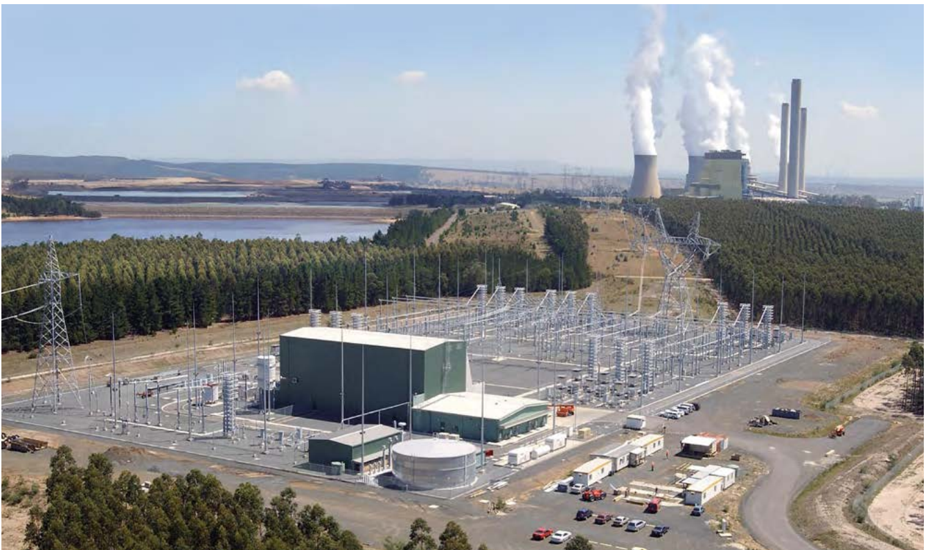
Fig. 2.2-77b, c: 400 kV HVDC Basslink project in Australia (monopole transmission line)
