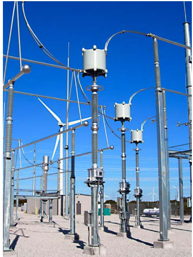
Fig. 4.2-33: Line traps
