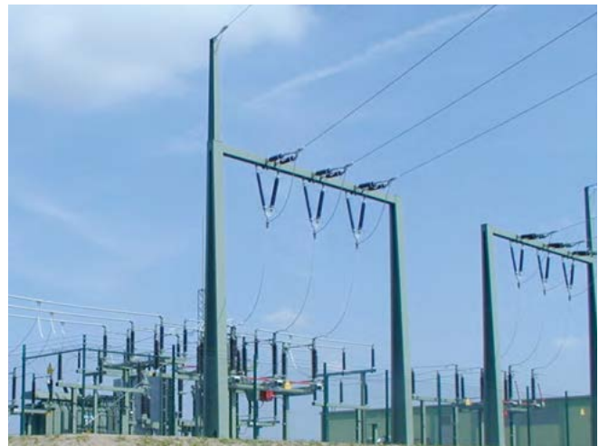
Fig. 3.1-12: H-arrangement, 110 kV, Germany
