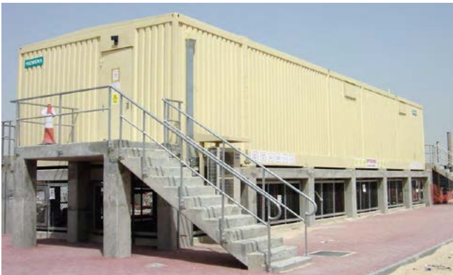
Fig. 2.4-5: E-house for Oil&Gas in Qatar
