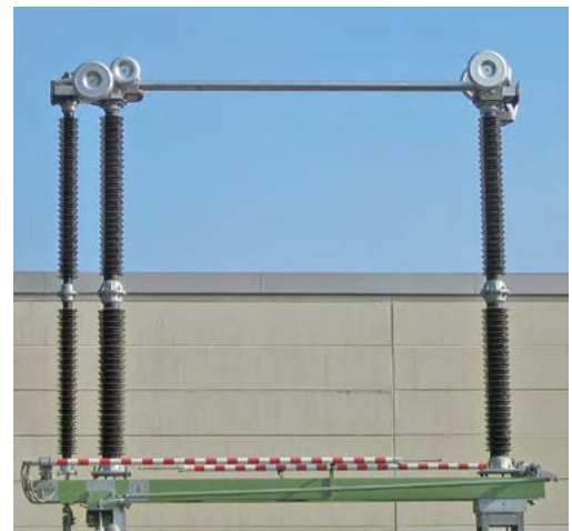
Fig. 4.1-27: Vertical-break disconnector
