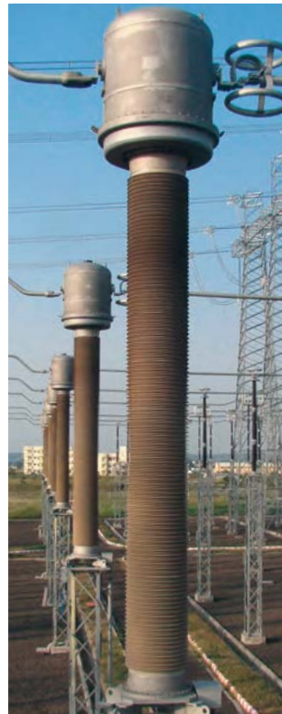
Fig. 4.2-13: 420 kV gas-insulated current transformers
