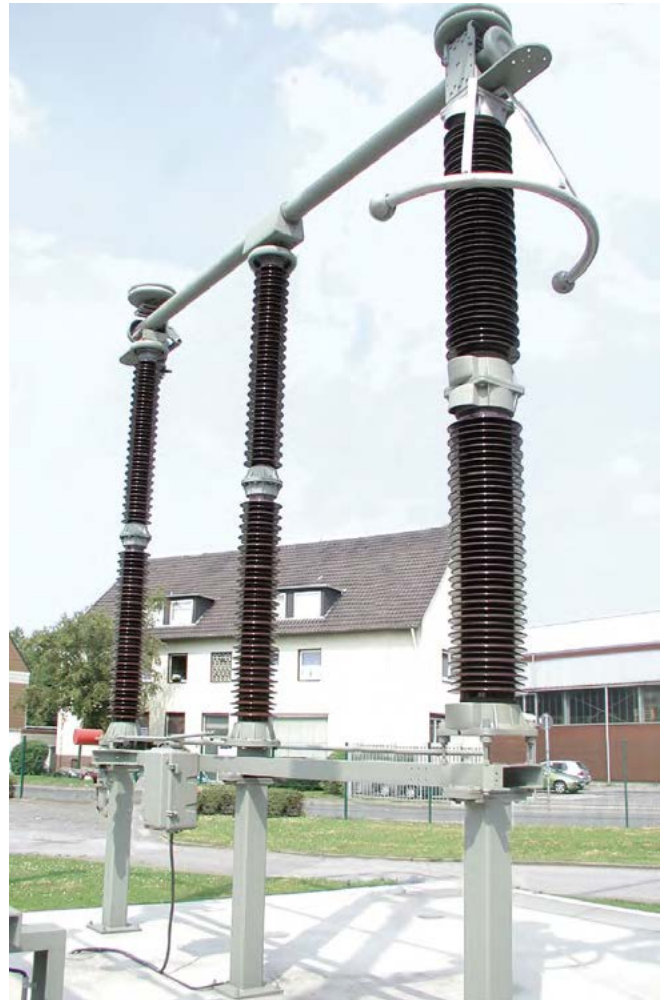
Fig. 4.1-28: Double-side break disconnector with integrated surge arrester
