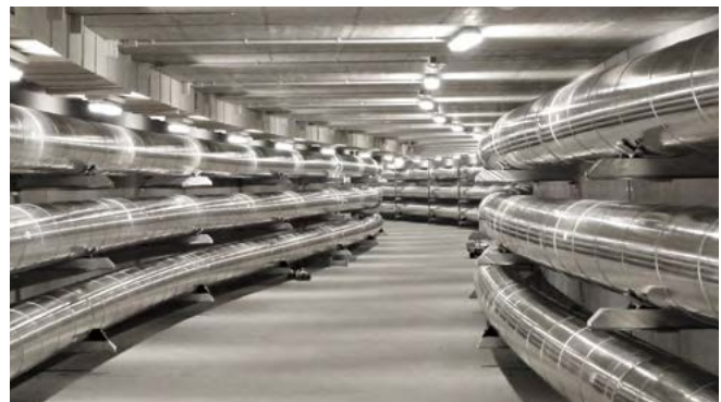
Fig. 2.2-46: GIL tunnel installation, Munich, Germany
