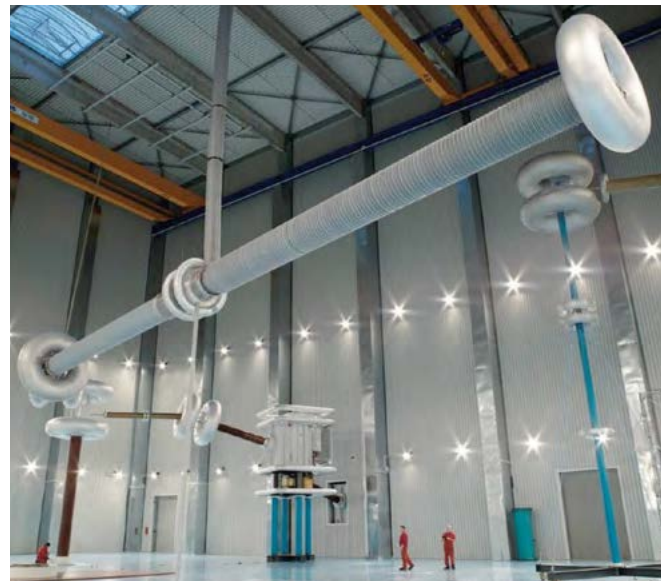
Fig. 2.2-4: A 20.8 m long wall bushing is required in order to connect the 800 kV terminal of the indoor thyristor valves to the outdoor HVDC equipment and overhead line
