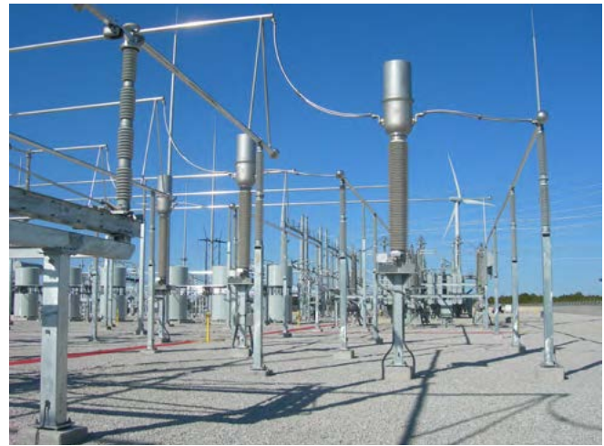
Fig. 4.2-21: 362 kV gas-filled combined instrument transformer
