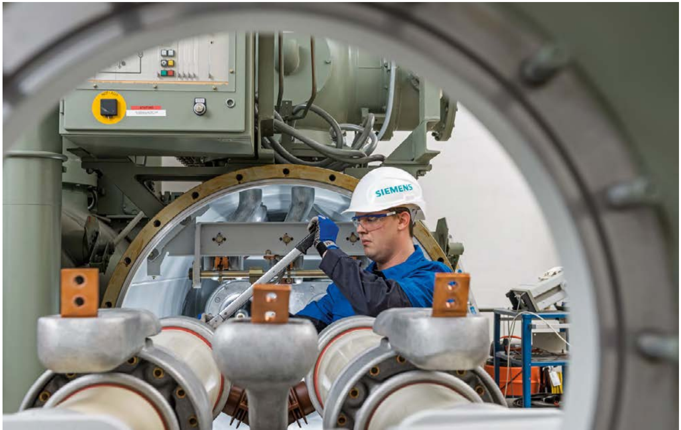
Fig. 10.3-2: Maintenance works on a HV GIS 8DN8
