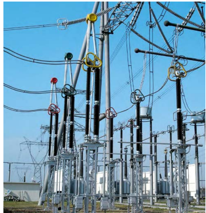
Fig. 4.1-29: Knee-type disconnector
