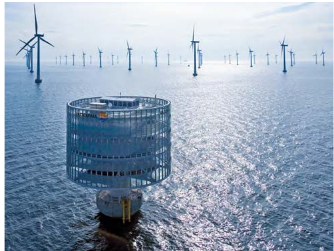
Fig. 2.2-30: 2007 110 MW Offshore Wind Farm Lillgrund, Sweden
