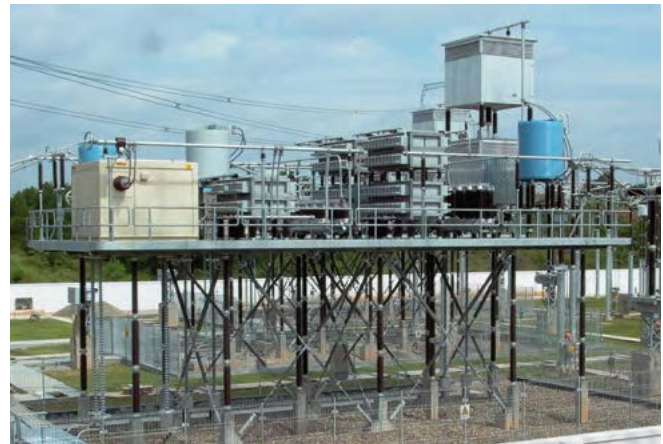
Fig. 2.2-22: View of a TCSC system
