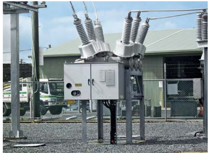
Fig. 4.1-11: SPS2/3AP1 DT 72.5 kV
