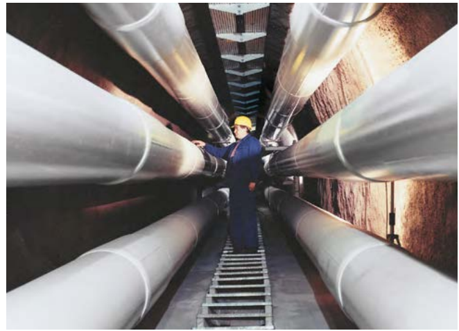
Fig. 2.2-39: GIL arrangement in the tunnel of the pumped-storage power plant in Wehr, Southern Germany (4,000 m length; in service since 1975)
