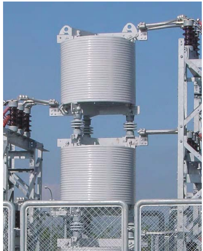
Fig. 4.2-34: 3-phase stacked current-limiting reactor
