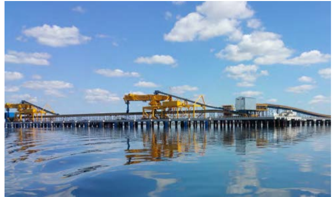
Fig. 2.4-9: E-house for the Nacala-a-Velha port in Mozambique
