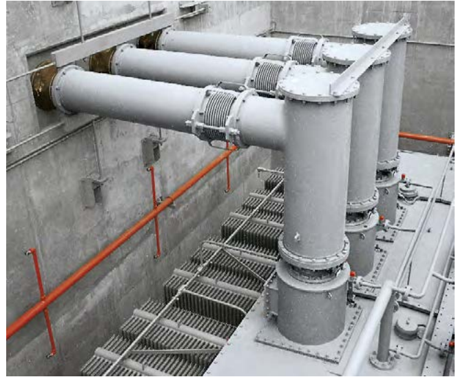
Fig. 3.1-46: Transformer termination
