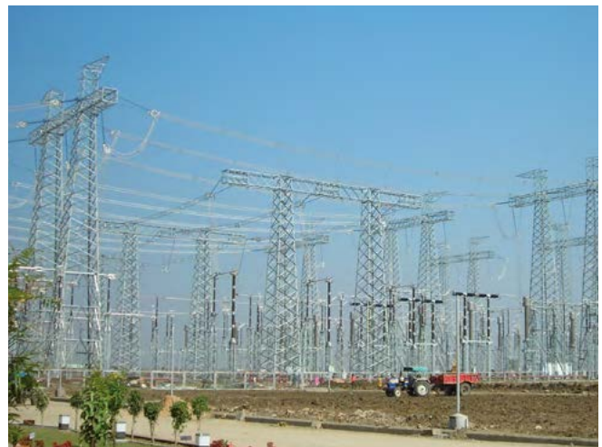
Fig. 3.1-22: One-breaker-and-a-half arrangement, 800 kV, India
