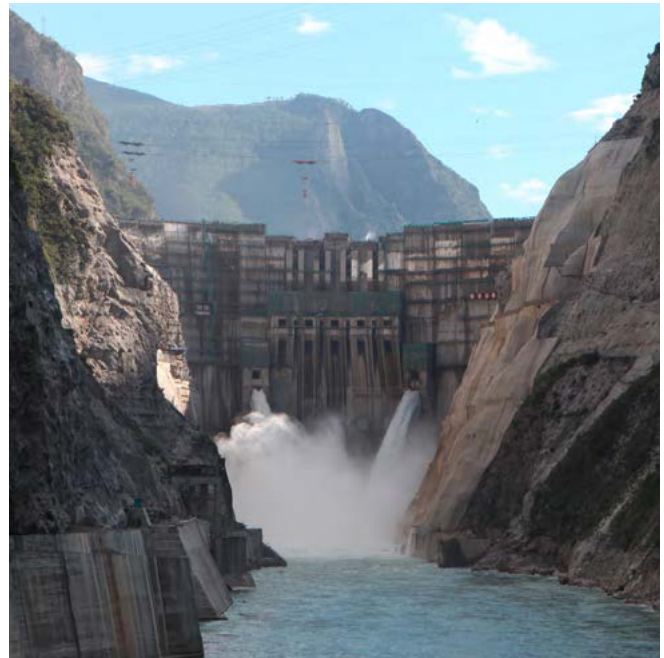
Fig. 2.2-52: Jinping, China, the world's tallest HPP dam
