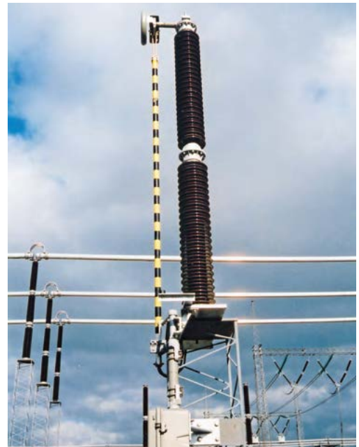
Fig. 4.1-30: Free-standing earthing switch
