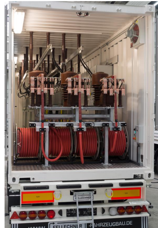
Interior view of a capacitor bank
